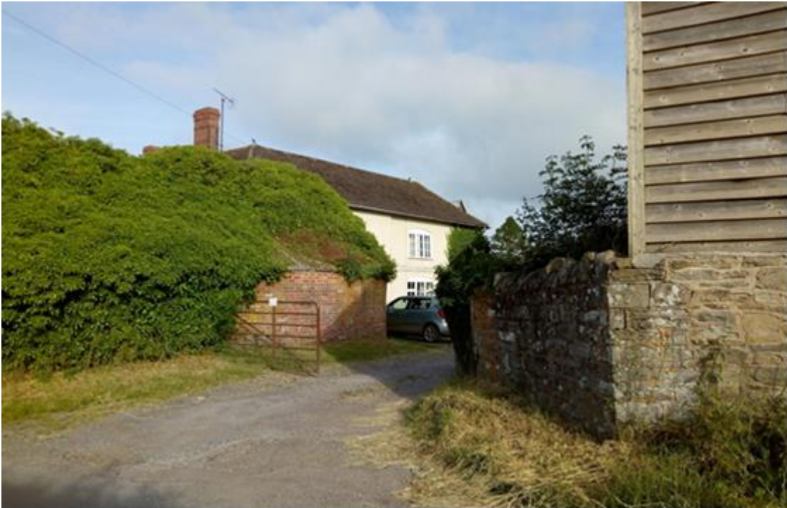
Figure 6: Grade II listed Woonton Farmhouse viewed from the east off Logaston Road
